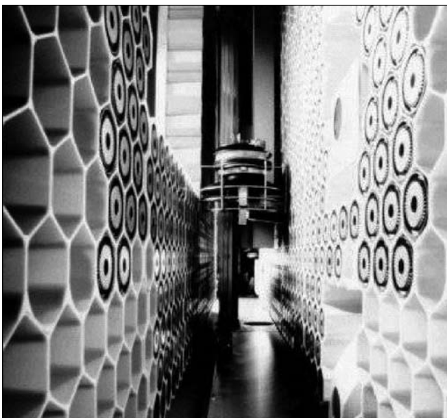
IBM Mass Storage System 3850 with 'Honeycomb Racks' 1974
